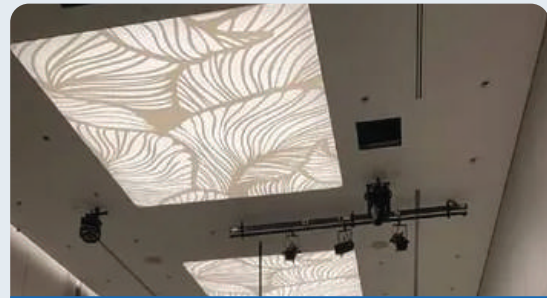
Stretch Ceiling Membrane
